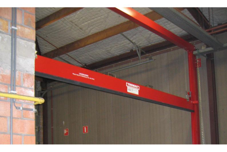
This TÜV and VdS-certified barrier rests above the door or gate opening when not in use. The barrier is manually operated via a chain and moves up and down within two U-shaped guides on either side of the passage. A counterweight provides weight compensation.
