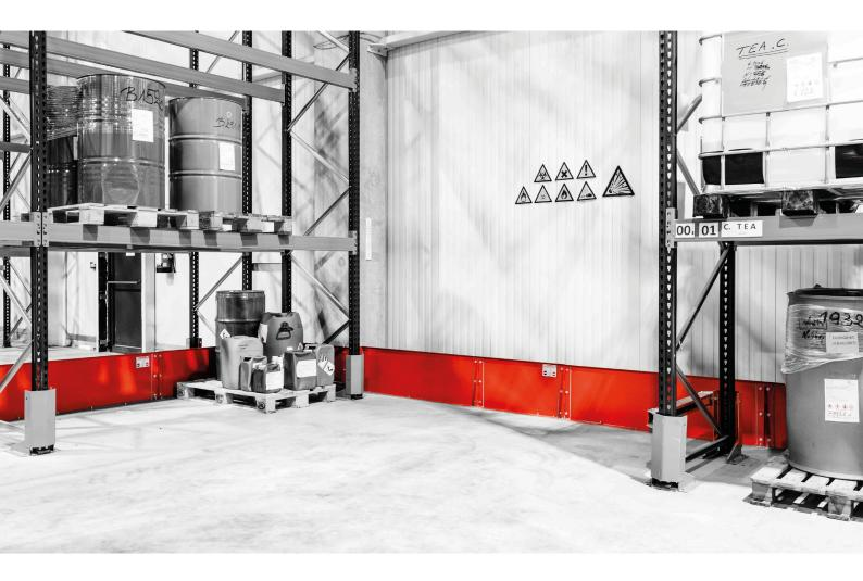
This permanent liquid barrier consists of an L-profile, securely bolted to the floor and walls. The barrier is installed and sealed watertight with caulking. It is placed around a designated area to create compartments or along the walls of a building, suitable for both short and very long sections.
