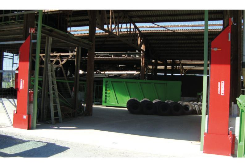
These TÜV and VdS-certified manual barriers are positioned on a base on both sides of the doorway (left and right).
