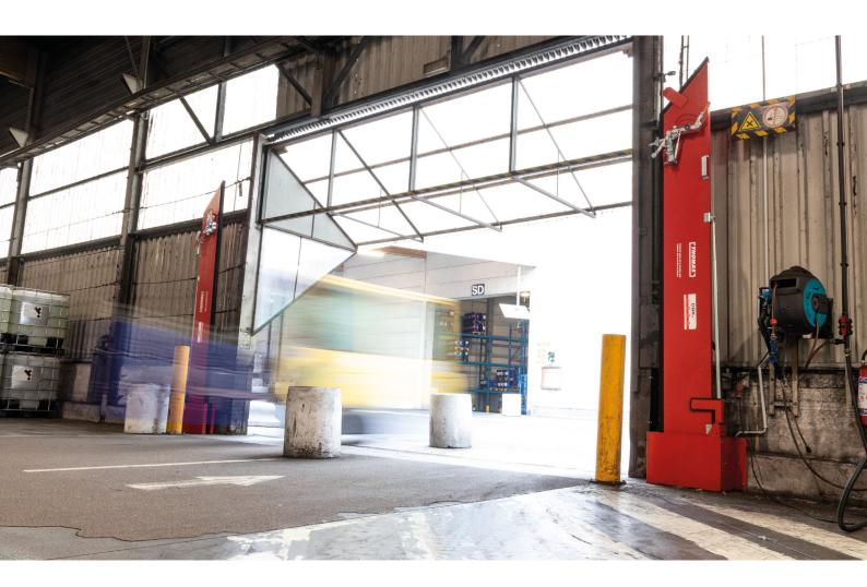
These TÜV and VdS-certified electromechanical/semi-automatic barriers are positioned vertically on both sides of the doorway (left and right). Each barrier is held in its upright position by an electromagnet.
